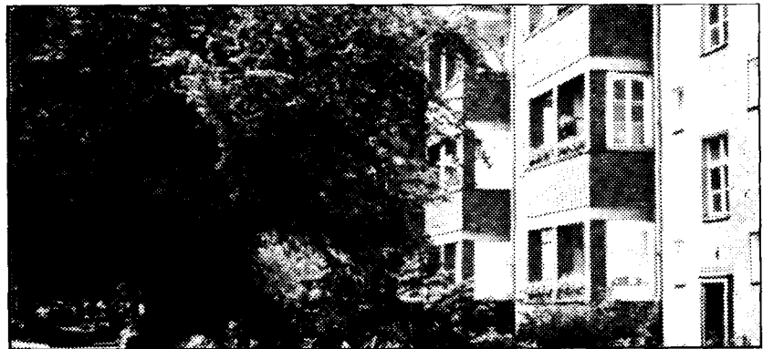
Figure 1.14 Suitable arrangement of vegetation: Directly in front of the building, the trees act as blockage against solar radiation, air filter against pollution, and reduce air velocity. Rising air is cool, moist and clean.
