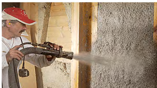
Implementation of cellulose flocks - © Thermofloc
