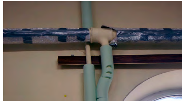
Insulation of pipework and valves - Pictures : Sylvie Rouche
