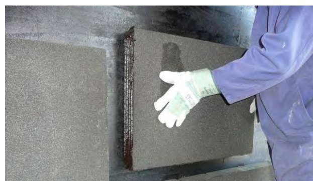
Implementation of cellular glass - © Foamglas
