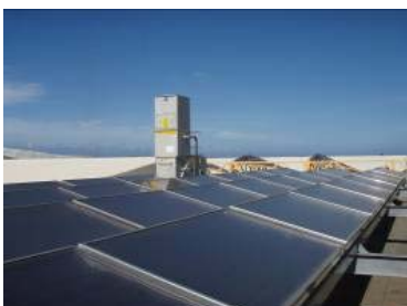
Solar cooling installation for a Tertiary building in Tropical climate (Source : TECSOL)
