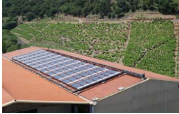
Solar cooling installation for a wine cellar in South of France (Source : TECSOL)
