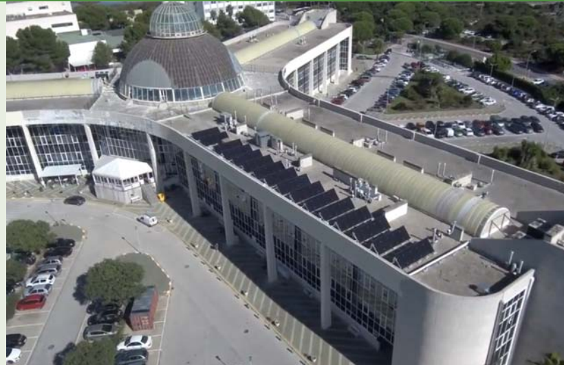
131 m 2 of uncovered PVT collectors in the south of Spain.
