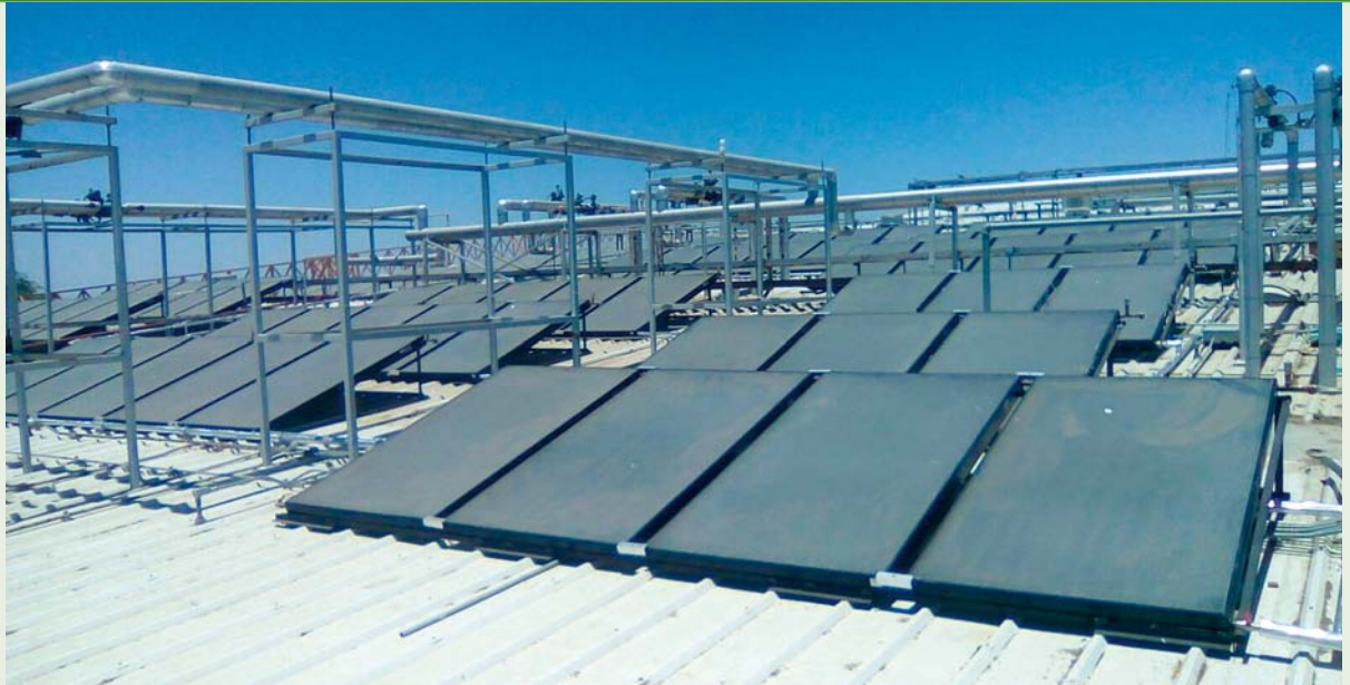
Flat-plate collectors for the food and beverage industry in Mexico.
