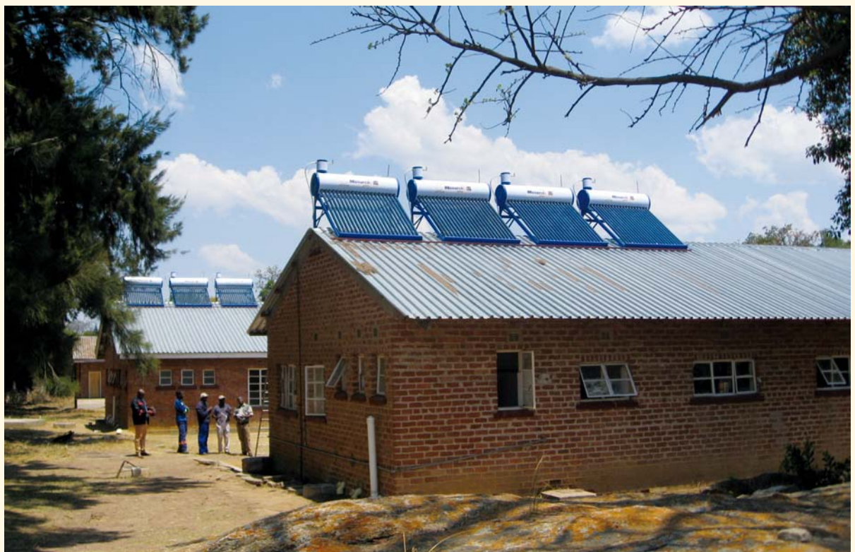
Demonstration system at Matopo Highschool in Zimbabwe with a collector area of 13 m 2 .
