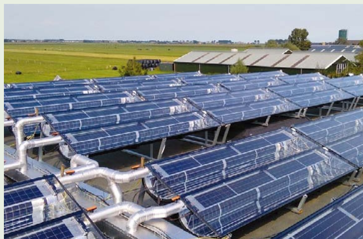
Low concentrating PVT collectors in the food industry in North Holland.
