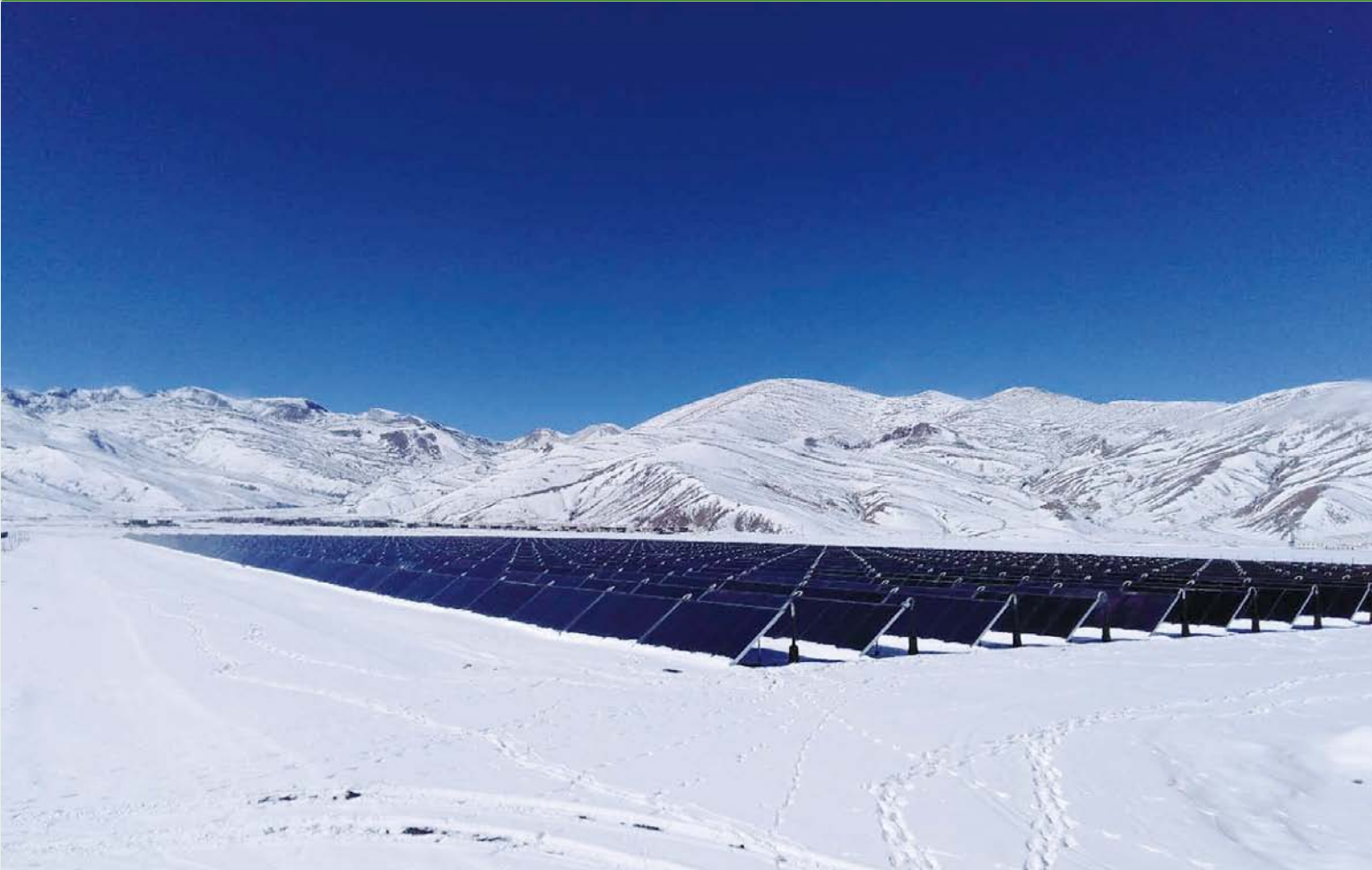
22,275 m 2 (15.6 MW th ) solar collector field covers more than 90% of Langkazi's heating needs in Tibet.
