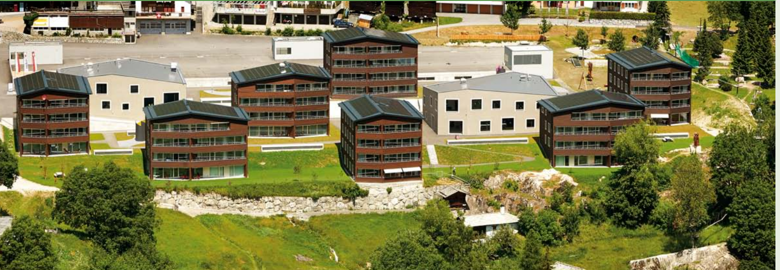
672 m 2 uncovered PVT collectors in Switzerland.
