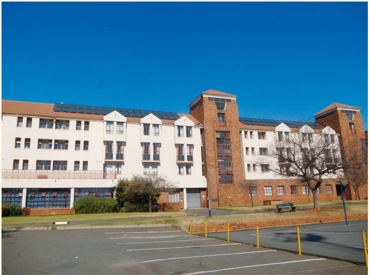
144 m 2 collector area at Barnato Hall student residences at the University of the Witwatersrand, South Africa.
