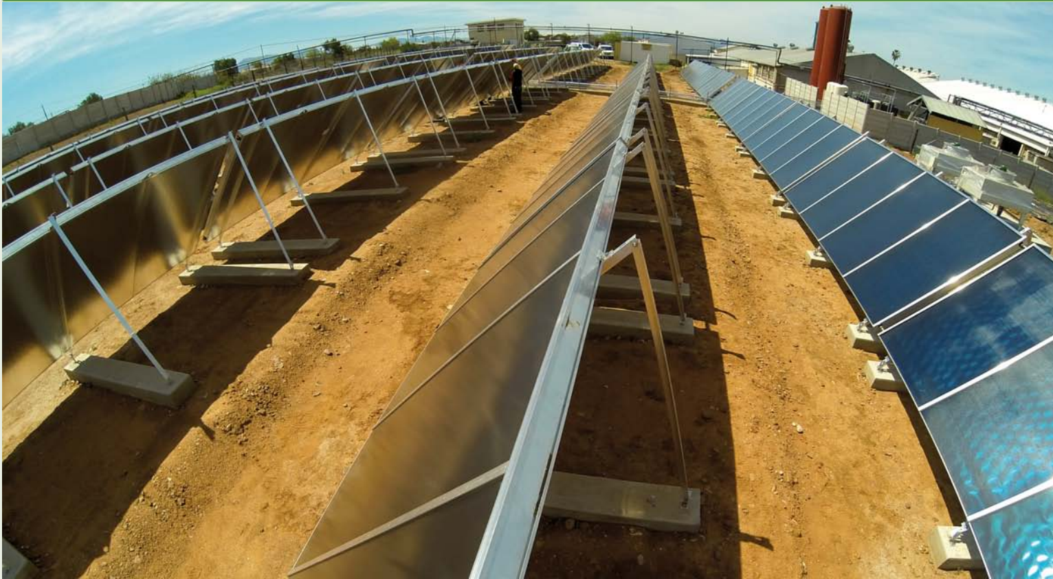
556 m 2 collector area provides solar process heat for Klein Karoo International Tannery in South Africa.
