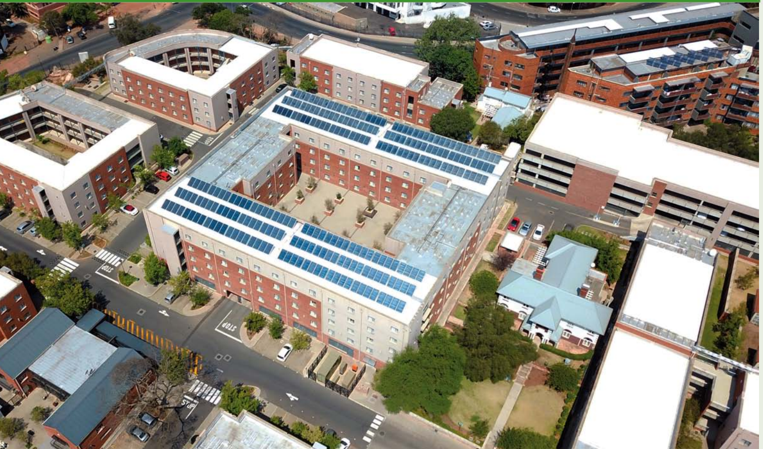
The WITS Junction system in the South African city of Johannesburg is the first solar district heating system in Sub Sahara Africa.
