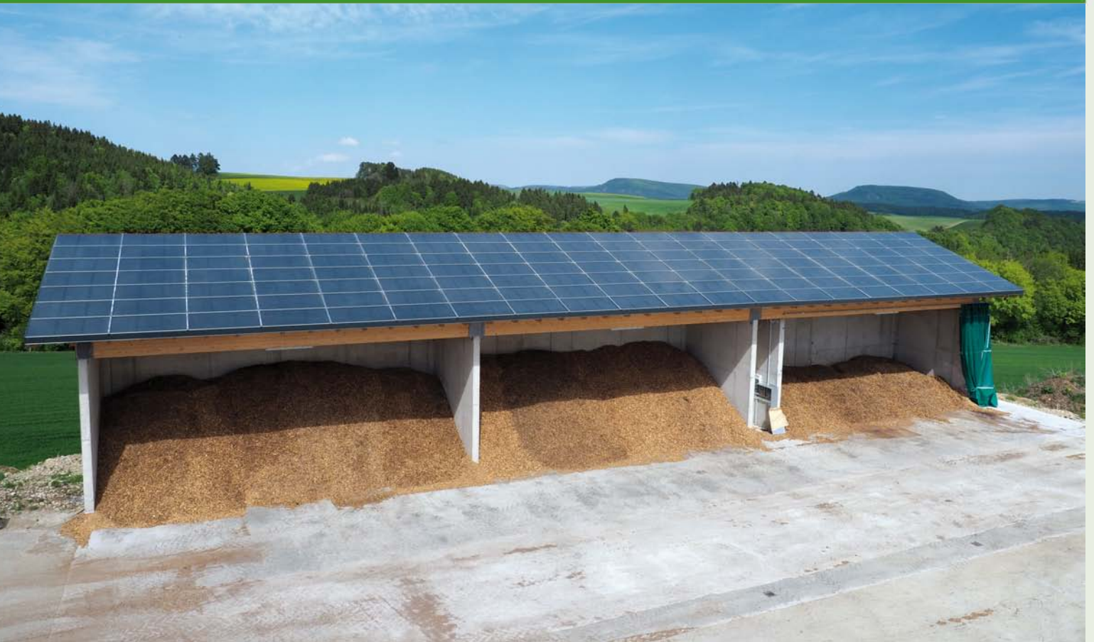
A 224 m 2 solar air collector field is used for commercial woodchips drying in Edlbach, Austria.
