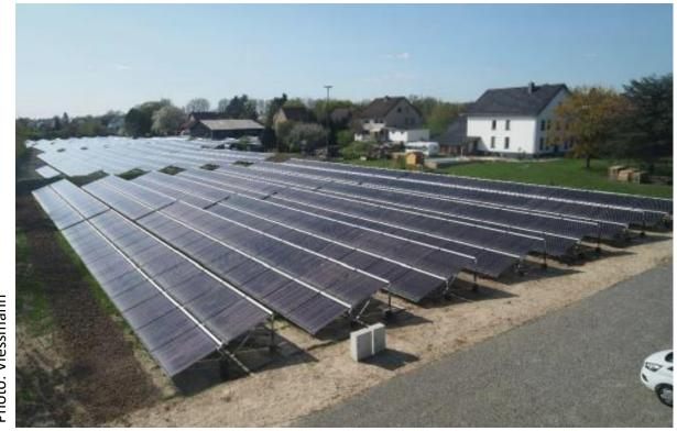
By adjusting the speed of the pumps in the solar circuit, this vacuum tube collector field delivers the required temperature of **90 °C** constantly.
