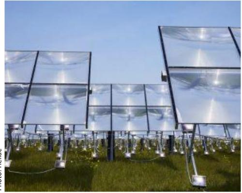
Concentrating collectors (Point Focus Fresnel) deliver heat at around **160** °C in Hørsholm, Denmark Photo: Aalborg CSP
