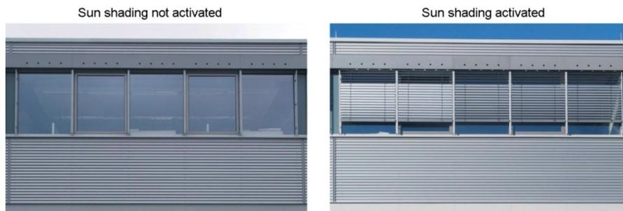
**Figure 17:** Photographs of the façade operating modes considered in a façade status-related, relative usable luminous exposure
