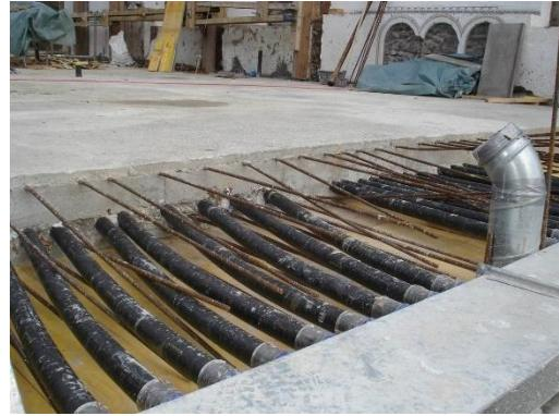
figure 40: Ventilation pipes in the floor © L. Carugo
