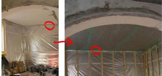
figure 15: © Vapour barrier on the walls and its connection to the vapour retarder in the ceiling (c)
