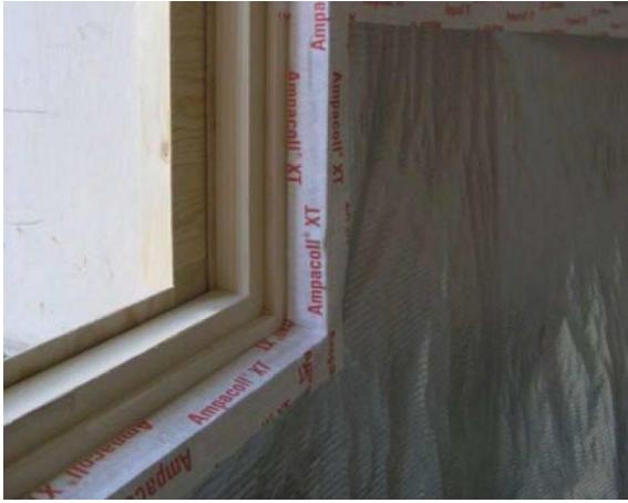
figure 13: Air-tight connection to the window frame (c)
