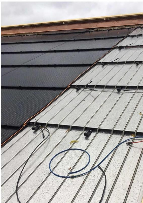
figure 107: PVT panels during works ©Studer
