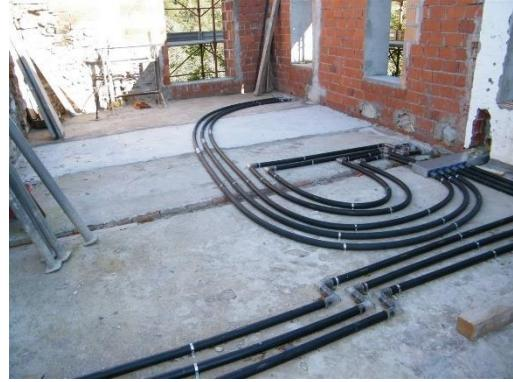
figure 41: Distribution in the floor © L. Carugo
