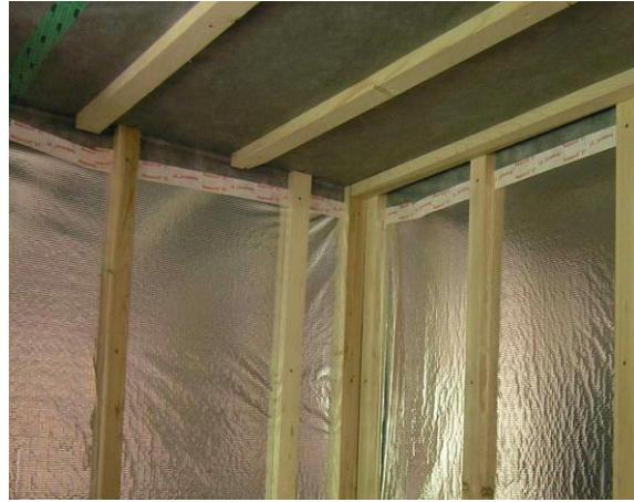
figure 14: Battens for installation layer, which avoids penetrating the vapour barrier with pipes and cables
