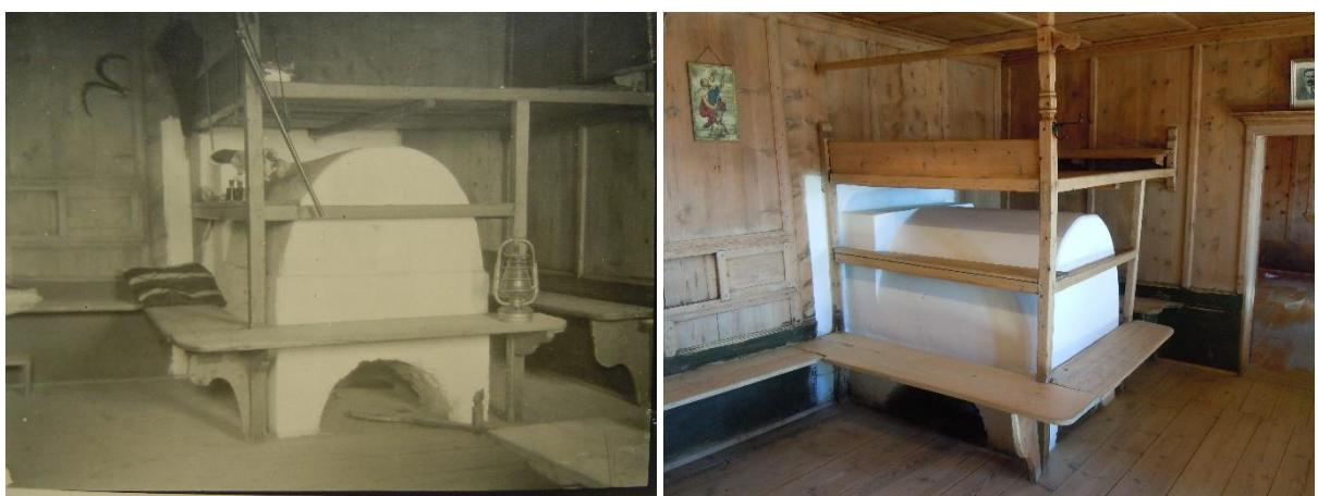
figure 63: Original tiled stove (left) and repaired (right) at Platzbon (Italy)
