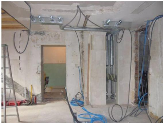
figure 23: Execution of pipes during the works ©V+P
