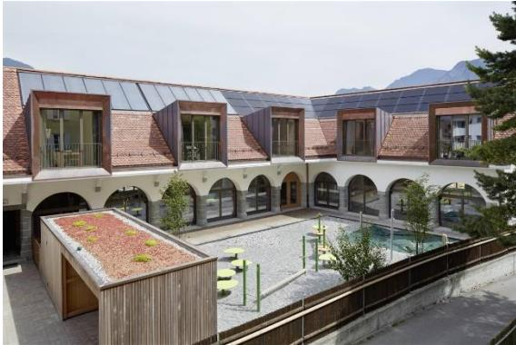
figure 91: Solar panels and PV integrated on the south front © Ralf Feiner, Malans
