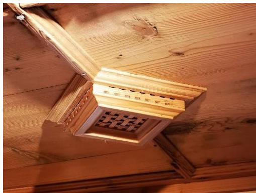
figure 114: Integration of an exhaust air opening in a typical suspended wooden ceiling as commonly found in Tyrolian farms. Source: Michael Flach
