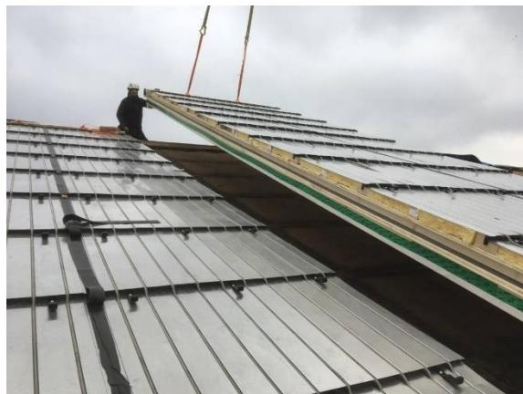
figure 108: PVT panels during works ©Studer
