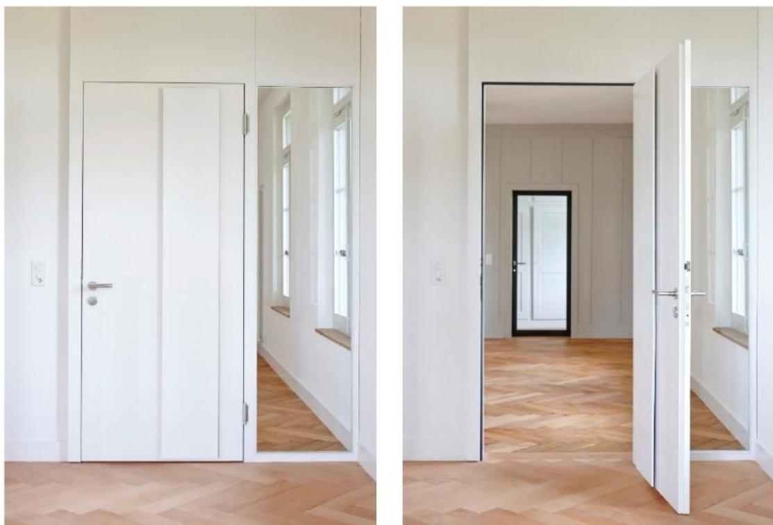
figure 19: Active overflow system as a so-called "Verbundlüfter" by the company Erich Keller integrated into the door leaf in the listed manor house Brünnengut in Bern (Switzerland).
