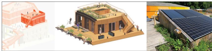
◀ The wood-based building of the VIRTUe team from the Netherlands can be used to add additional floor space to existing buildings. The roof is walkable and includes a PVT field plus a solar collector linked to the house's underfloor heating and cooling system.
