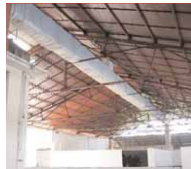
Duct work for the solar panels mounted under the roof at the moyu drying plant in China.
