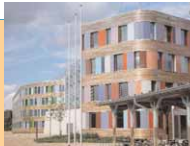
Germany's new Federal Office on Environment or Dessau is energy efficient and uses renewables including solar collectors and daylighting.
