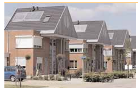
Typical installation of solar collectors on new buildings in the Netherlands.
