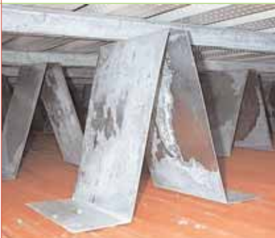
Metal "hats" hold perforated solar panel of roof and form the air space from which the solar heated air is drawn.
