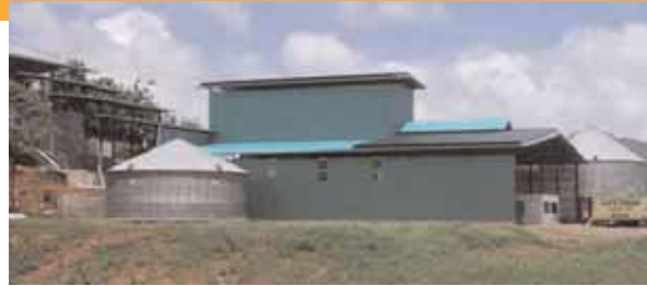
Panama coffee drying facility shows collectors installed on the lower and upper roofs.
