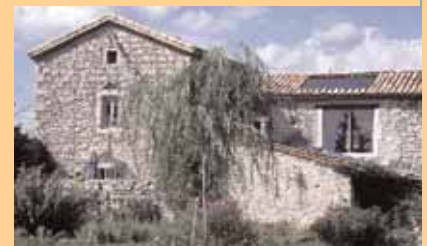
A French home with a roof integrated solar water collector.
