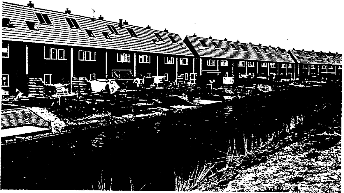
Photo 2. Domestic Hot Water System Demonstration in Alkmaar (NL-5)
