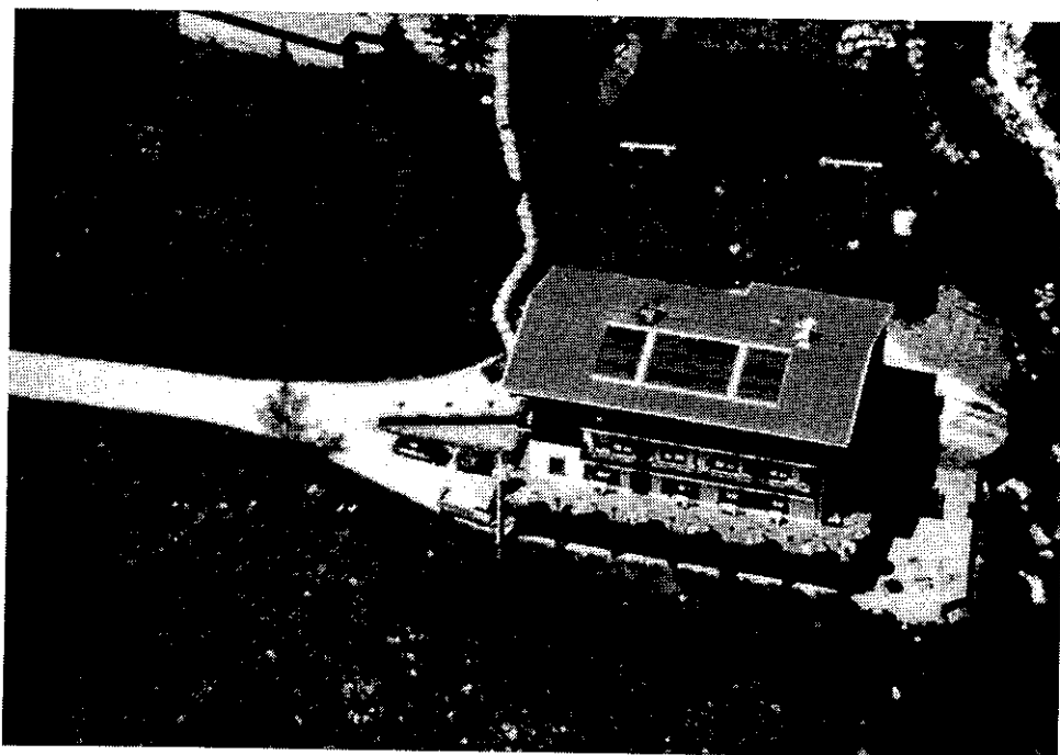
Fig. 1. Integration of solar collectors in buildings: example of a hotel.
