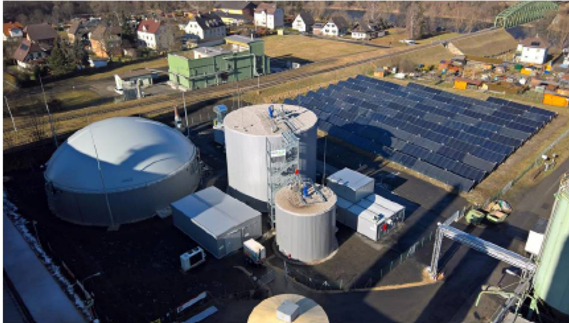
Process heat plant at Goess Brewery in Austria, 1 MW th installed capacity
